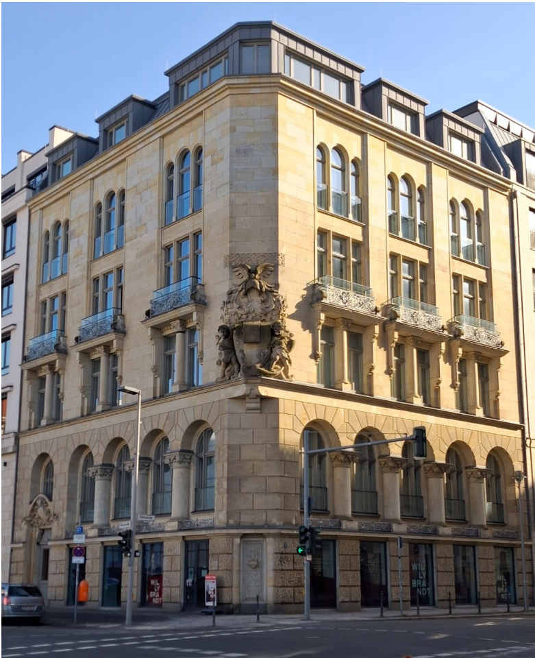
Figure 2 Behrenstraße 14–16, now Palais Theising. Source: private; photographer: Dörte Lerp.
